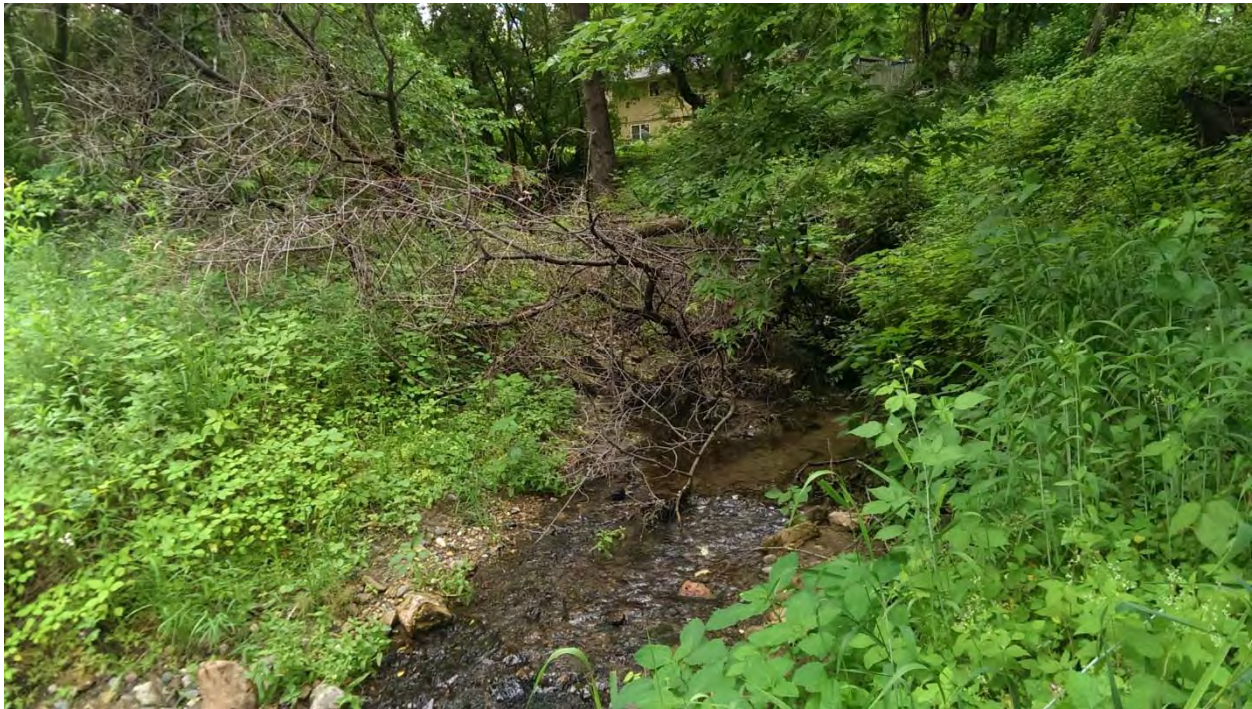
Photo 2: Stream section facing upstream directly behind garage (sudden drop-off on the right caused by recent erosion, new plant growth on the left, and a previously fallen tree caused by stream bank instability)
