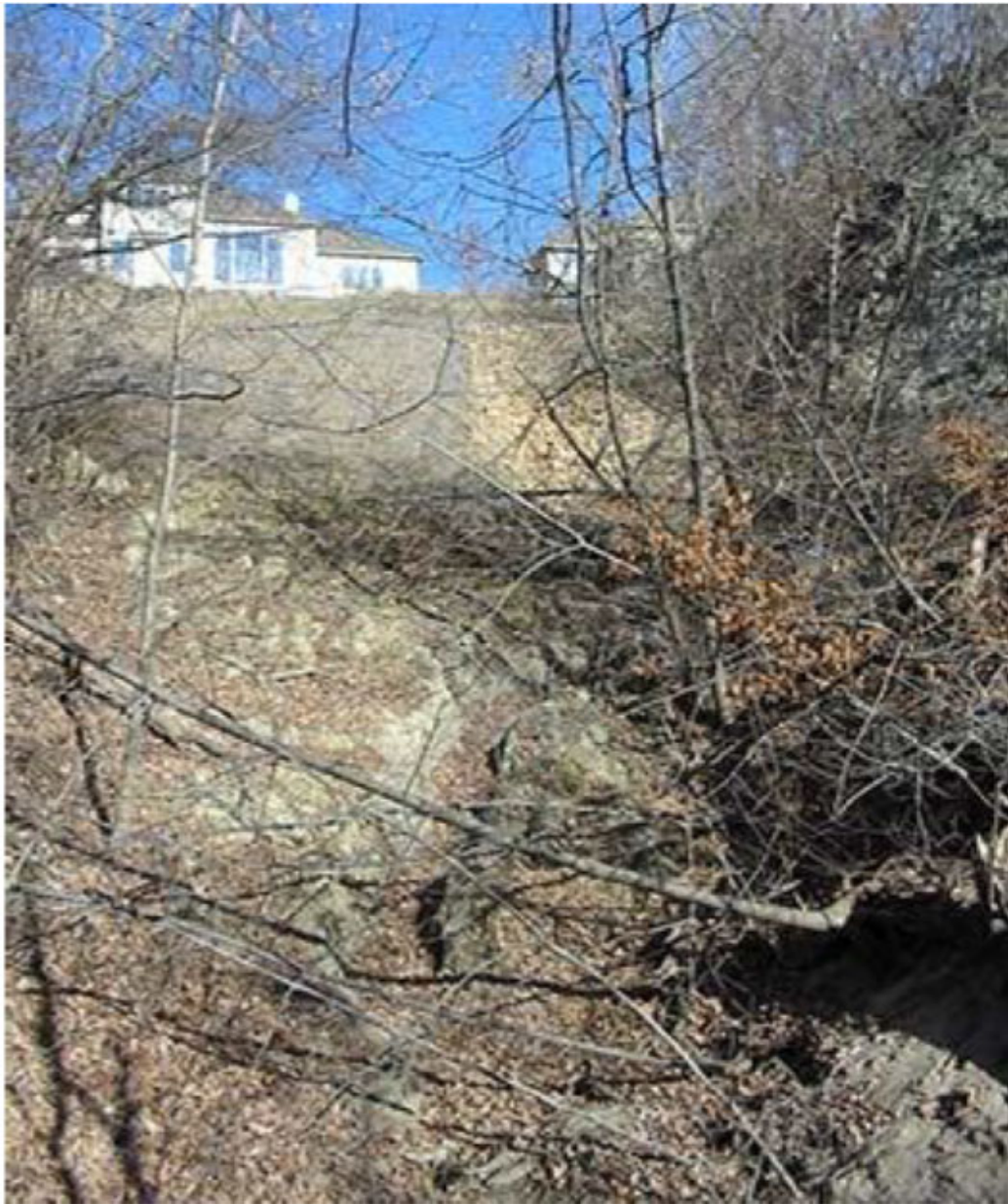
Figure 98. Photo of Site L434 from 2008 Inventory.
