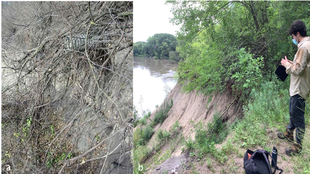
Figure 101. Progression of erosion at Site L275 from 2008 (a) to 2020 (b).
