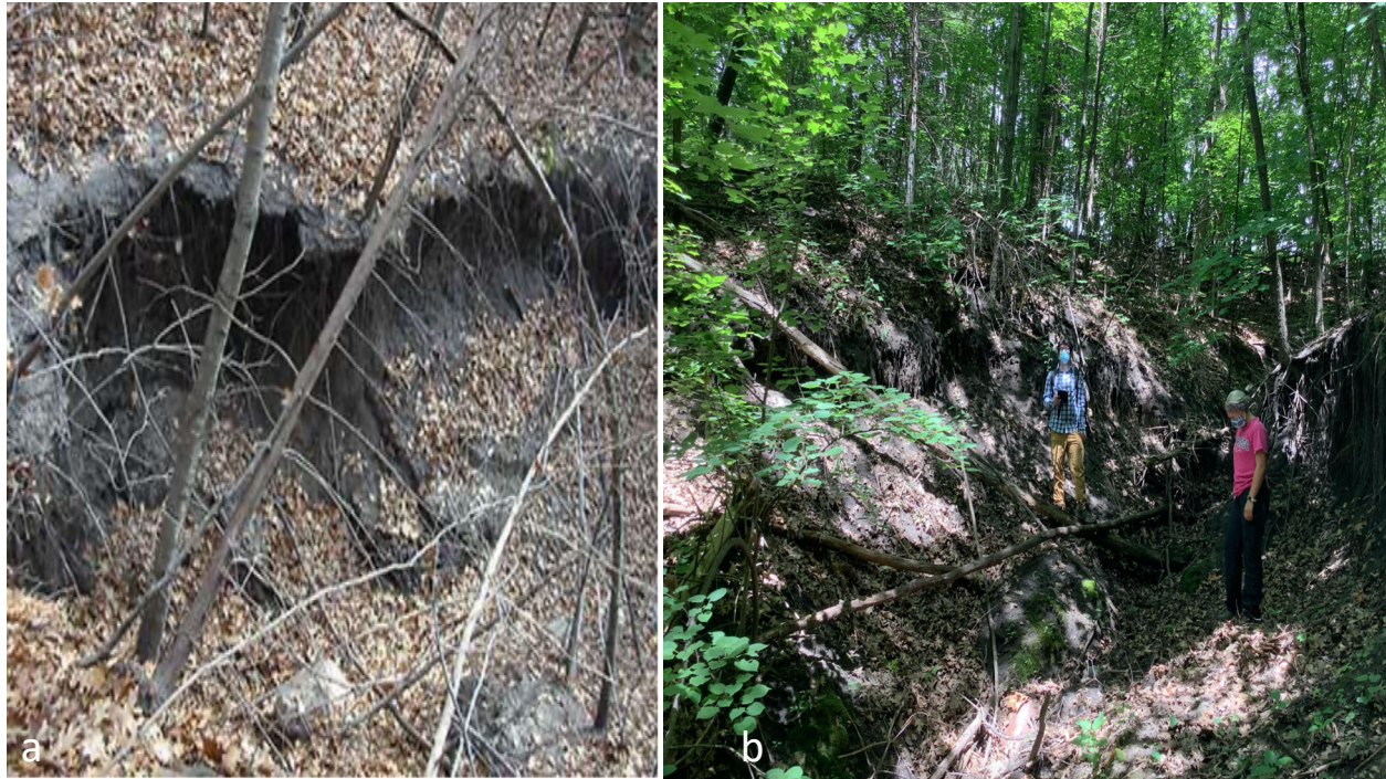
Figure 51. Photo 'a' is an image of L128's channel and banks taken in 2008; Photo 'b' is an upstream view of L128's channel taken in 2020.
