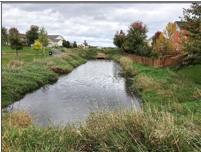
Photo 5: excavated detention pond, view east.
